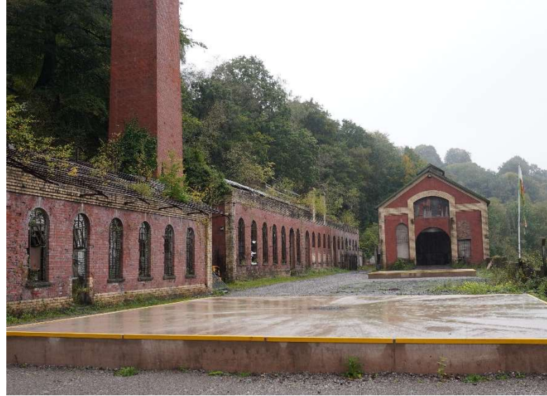
View north on site's upper level, with mine caps, workshop and north winding house in view
